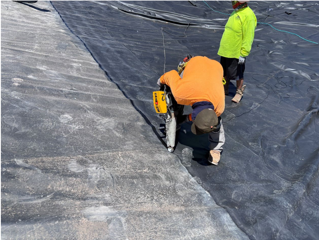
Photo 9: Extrusion welding the new liner to the existing liner
