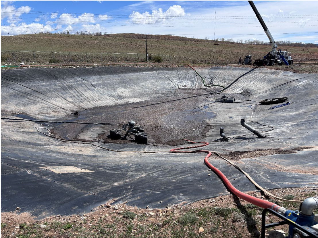
Photo 1: View of the mostly dewatered activated sludge lagoon
