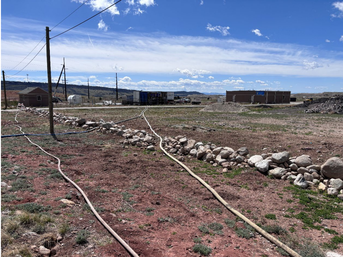
Photo 3: Hoses pumping decant liquid to sewer manhole at the wastewater plant influent pipeline
