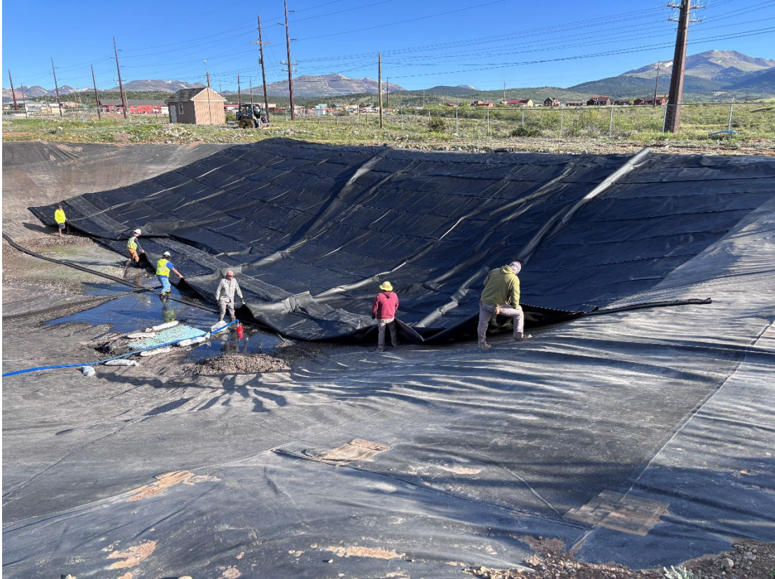
Photo 7: Simbeck Liner pulling new RPP liner sheet down into the lagoon
