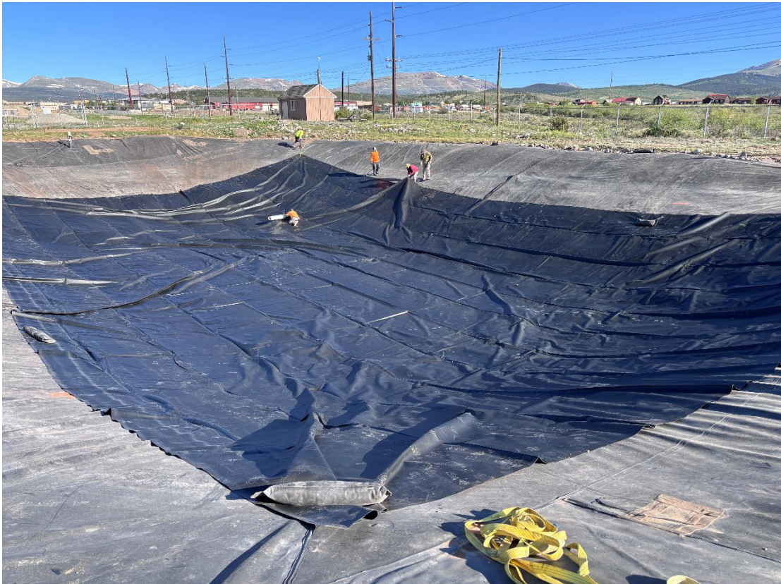
Photo 8: Liner in place and ready for cutting to fit and welding
