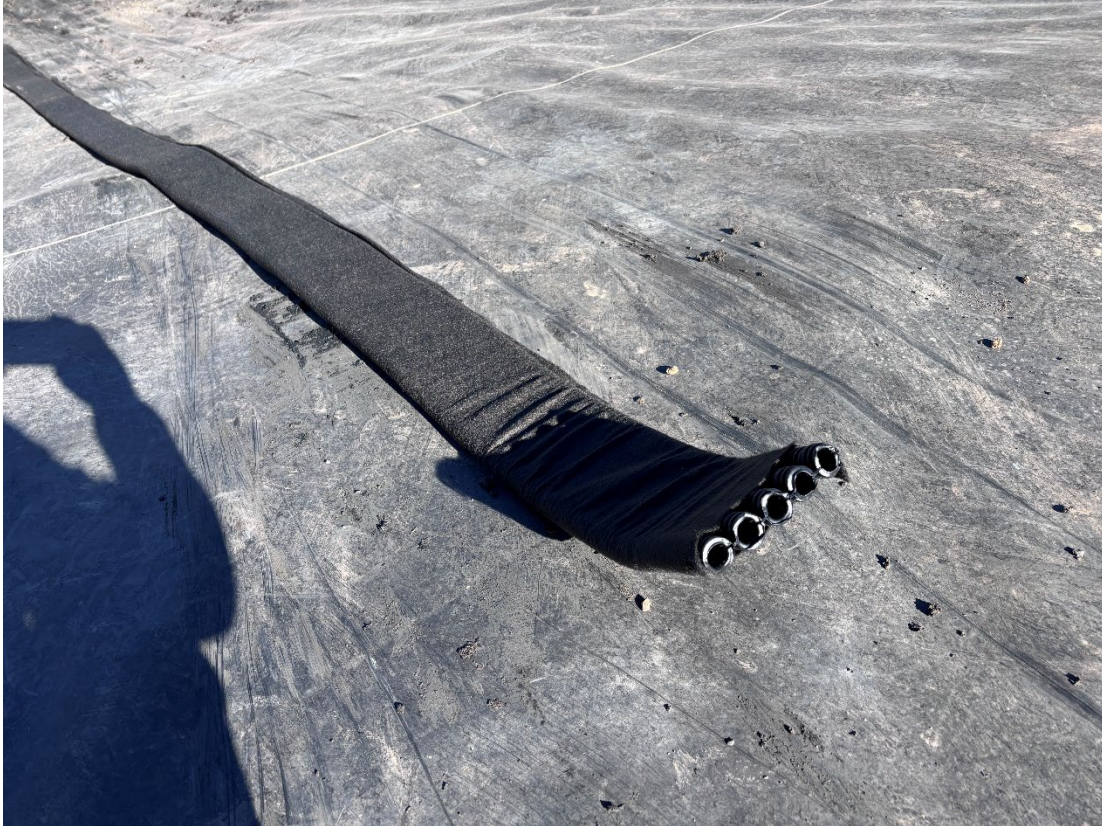
Photo 6: View of perforated vent stripping
