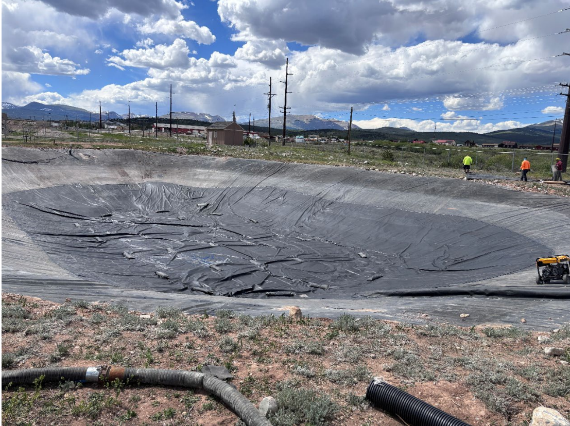
Photo 12: Completed liner repair
