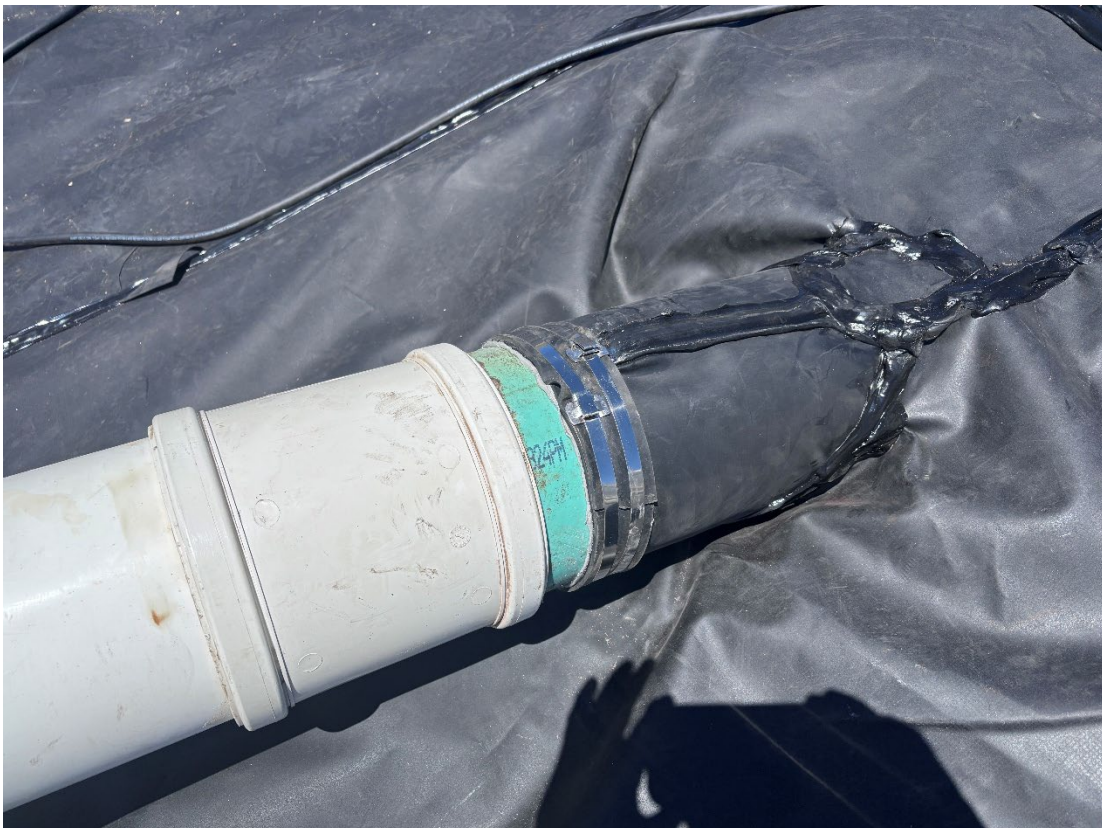
Photo 10: Finished liner boot installed at a pipe penetration
