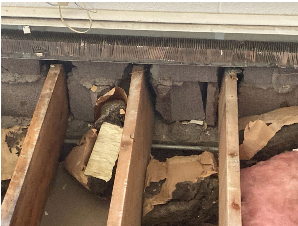
Main Street Load Bearing Wall – Old Floor Joists
