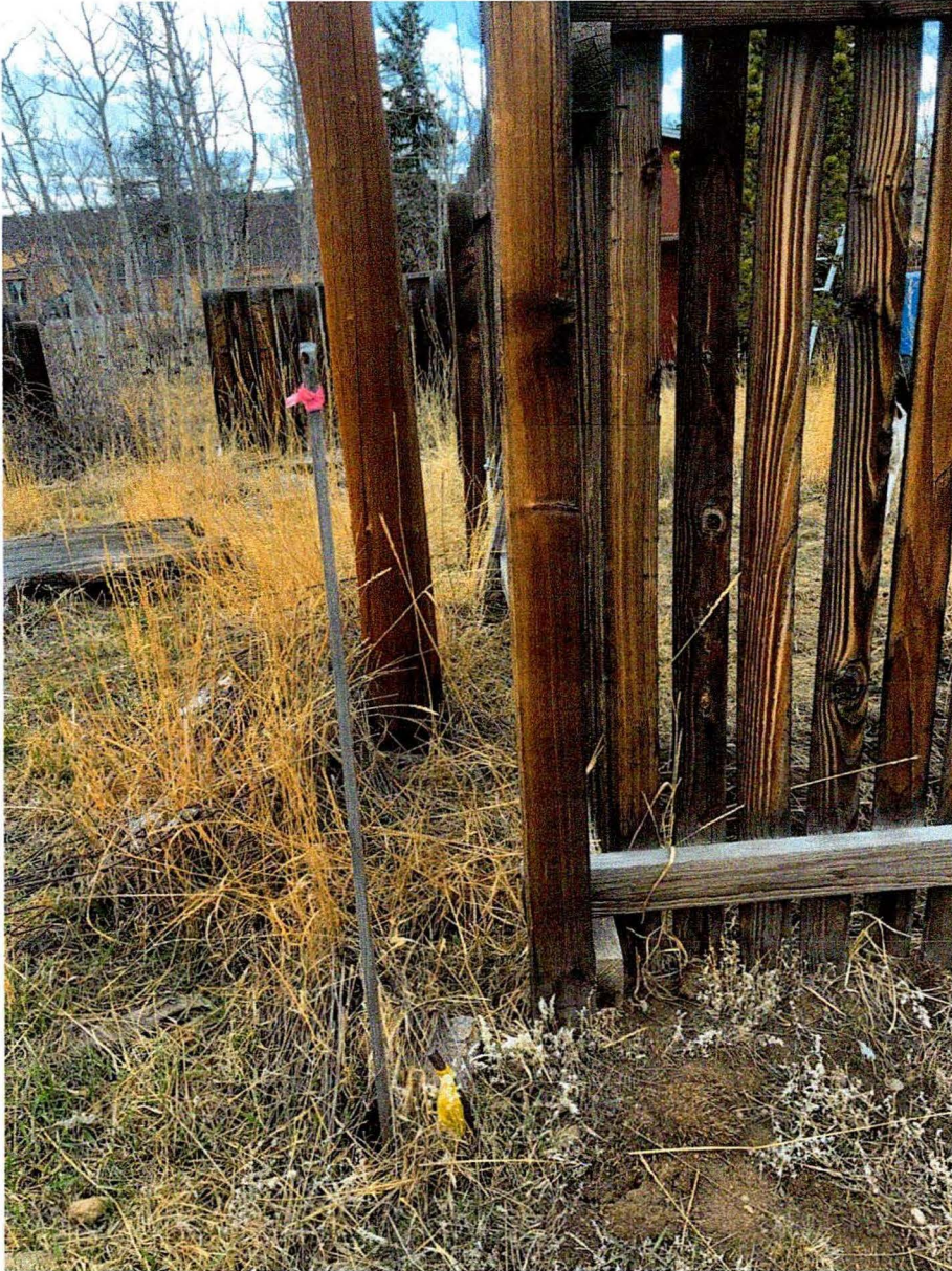
Southeast corner of property. The survey stake and metal marker indicate that the fence line is about a foot inside our property line at this time.
