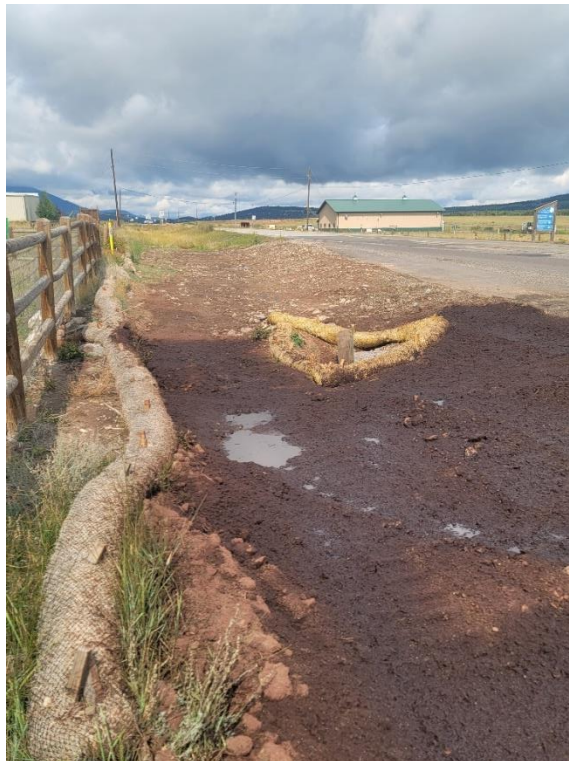
Photos 1-3 – CDOT ditch and 24" concrete culvert (under construction)
